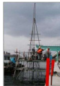
Core Drilling
