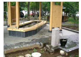
Foot Bath Facility
