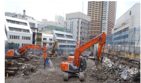
Demolition Work in Urban Area
