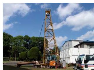
Hot Spring Drilling
