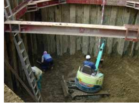
Removal of Contaminate Soil
