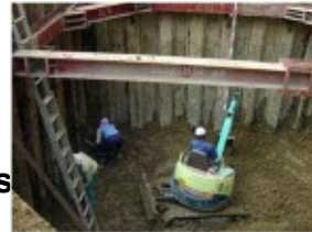
Removal of Contaminate Soil
