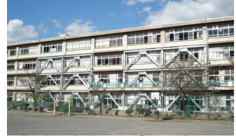
Design of Vibration Control Braces
